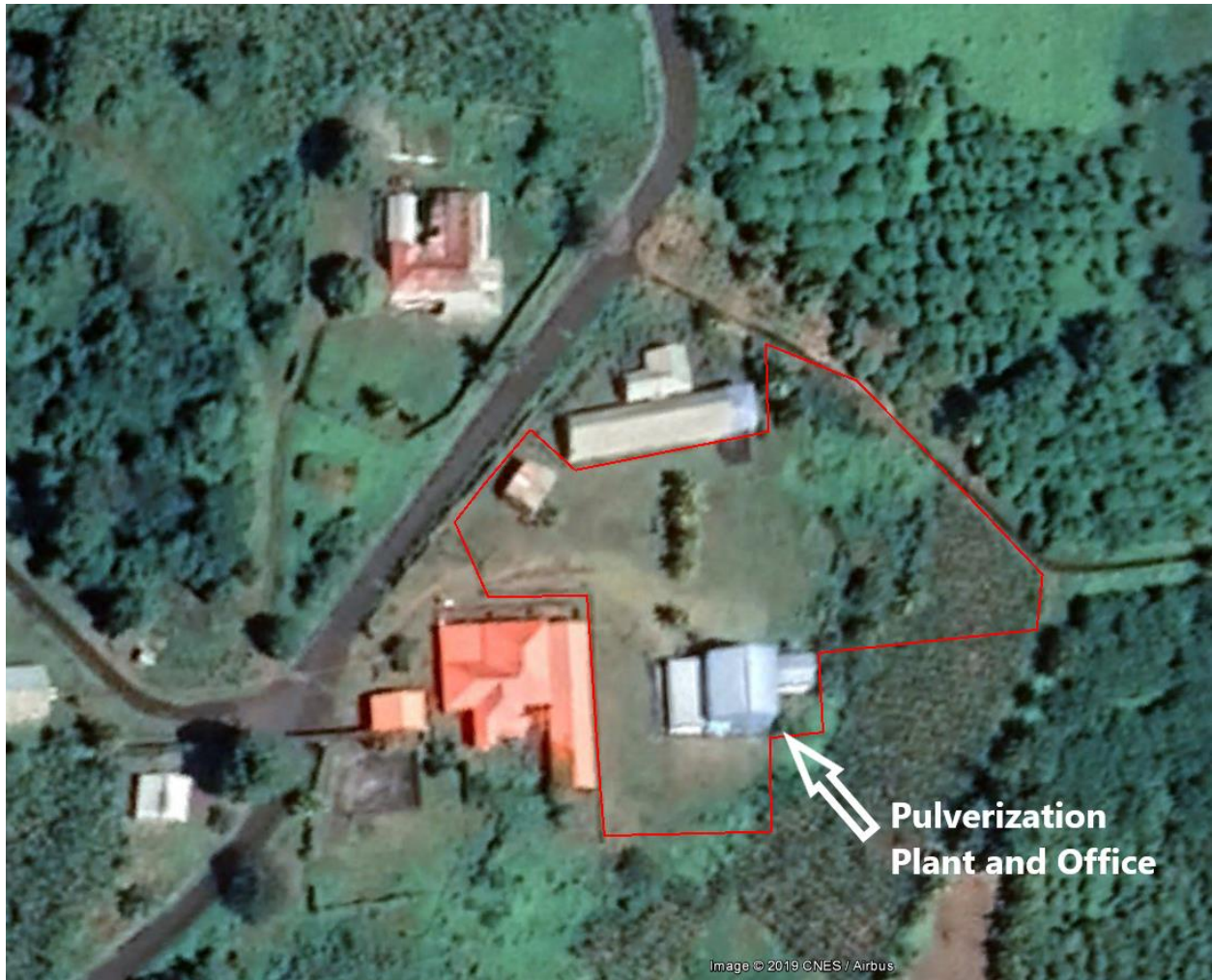
Site Photograph showing existing pulverization plant and other buildings on site
